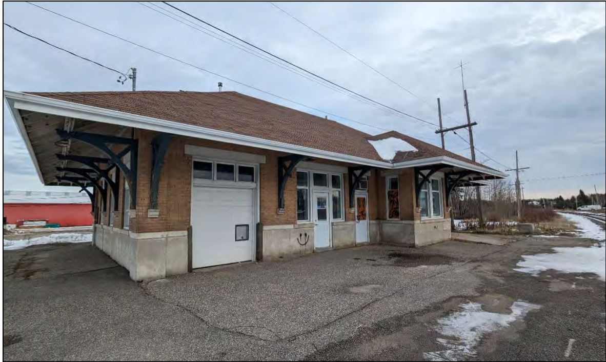
Photo 2: Site building facing South
