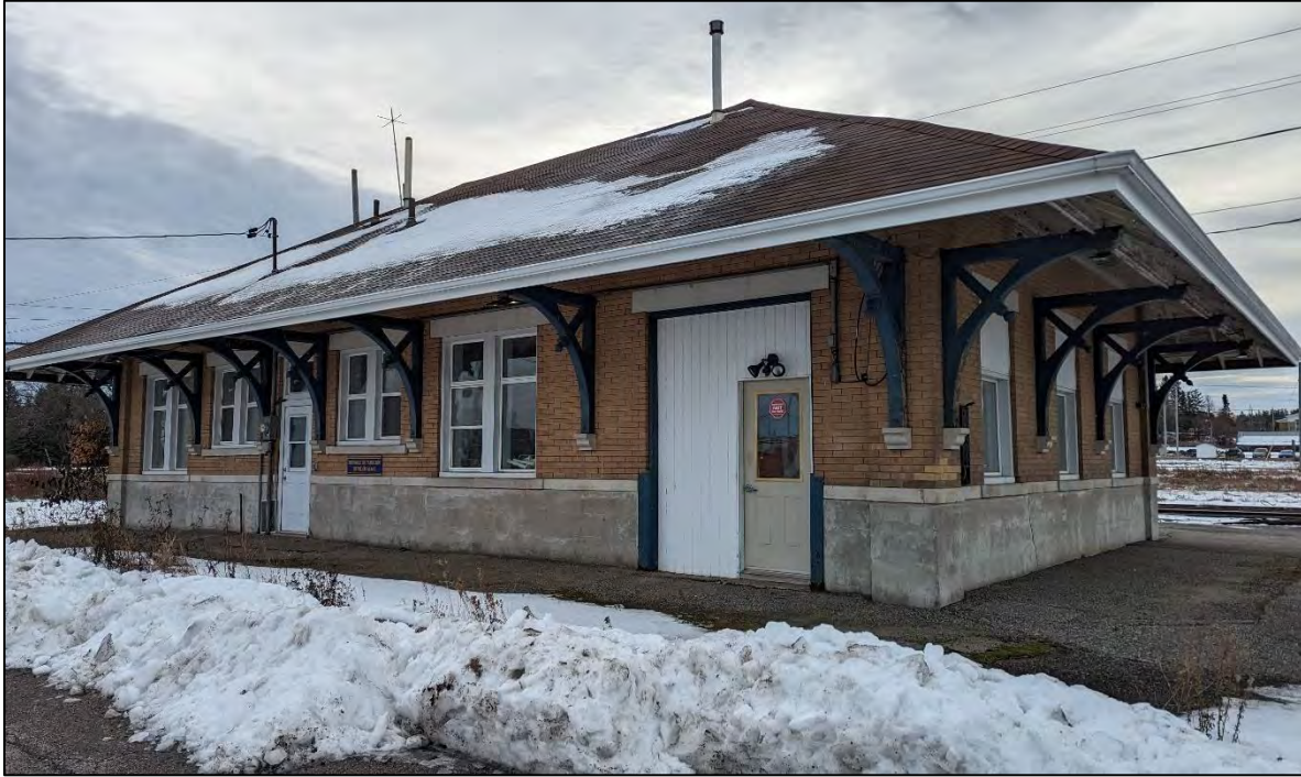
Photo 1: Site building facing North.
