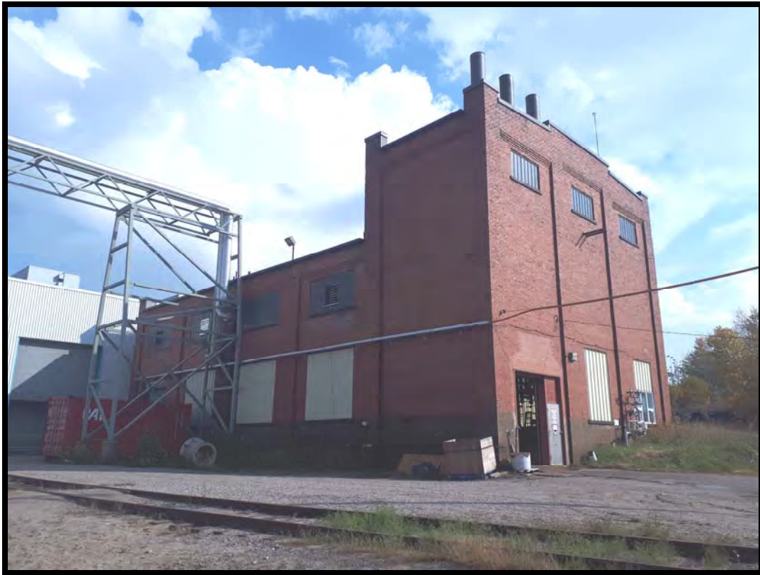
PHOTO # 1 POWER HOUSE
