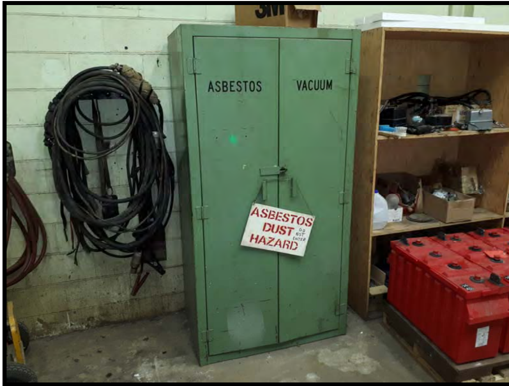
PHOTO # 43b Asbestos-containing materials within storage cabinet in Car Shop – Room 117
