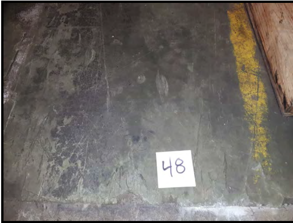
PHOTO # 31 Sample # ONR – 48 : Non-asbestos Roll Vinyl Flooring in Diesel Shop - Room # 12.
